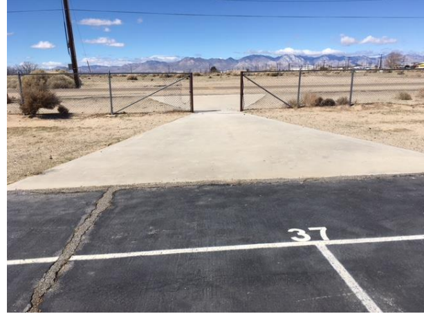
MJH58 – remove concrete apron out to road; remove MMS perimeter fence; pulverize asphalt court; import clean fill dirt; smooth finish grade; no ponding
