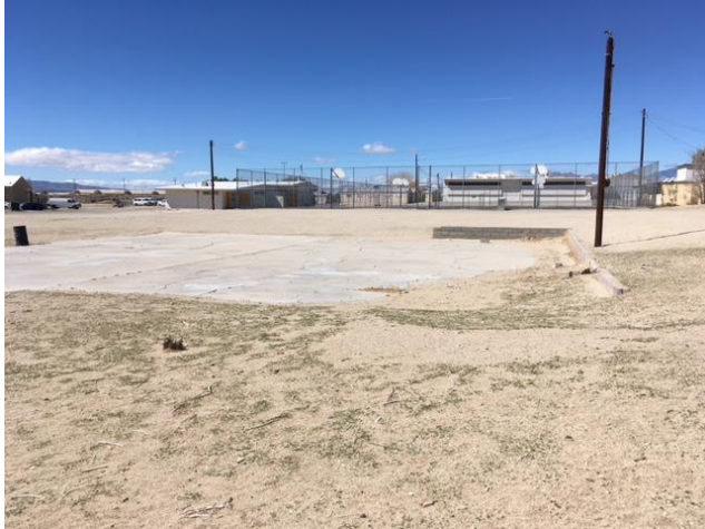
MJH56 – remove concrete slab, retaining wall, footing, wood pole, gymnastic pipes & footings, bf/compact
