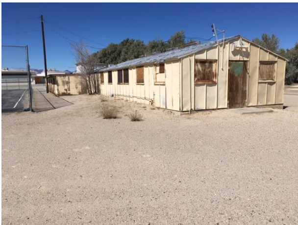
MJH54 – demolish & remove from site metal building, SOG, footings, cut & cap water, sewer & gas 5' from building; remove power pole, bf/compact; import clean fill dirt, smooth finish grade area with adjacent area of MJH 52 (track & field); no ponding in finish grade
