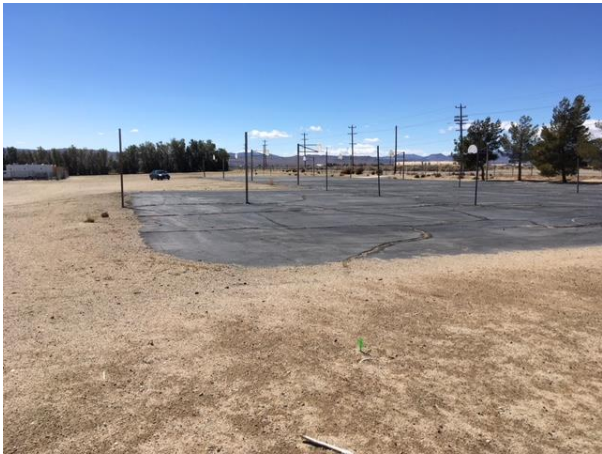
MJH58 – pulverize asphalt court and smooth grade; remove concrete structure & bench; import clean fill dirt; smooth finish grade; no ponding
