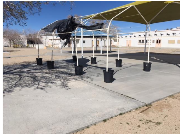
MJH33 – demolish & remove temporary pipe shelter
