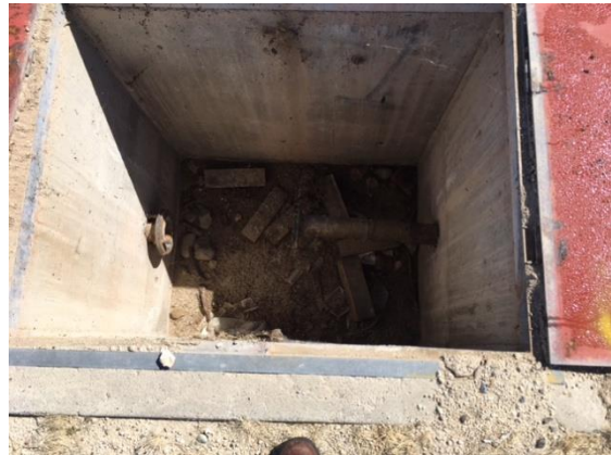
Remove MMS perimeter fence, posts, bf/compact
