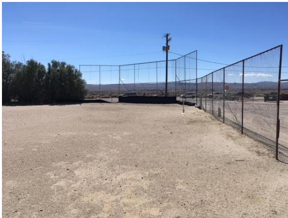
MJH55 – remove backstop, fence, posts, bf/compact
