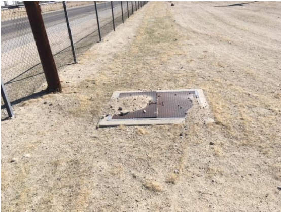
MJH52 – remove concrete vault, cap lines, bf/compact
