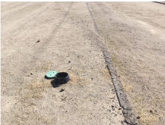
MJH52 – remove valve & box, cap line, bf/compact (typ)
