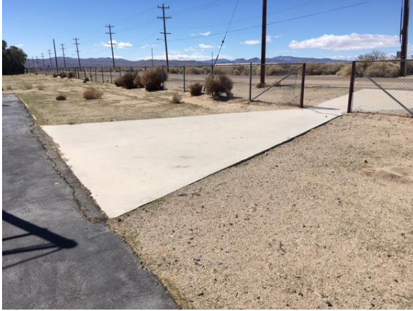
MJH58 – remove concrete apron out to road; remove MMS perimeter fence; pulverize asphalt court; import clean fill dirt; smooth finish grade; no ponding
