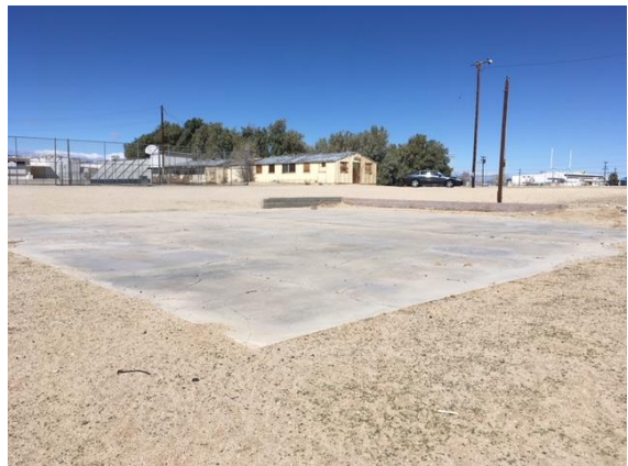
MJH56 softball field west – remove concrete slab, retaining wall, footing & wood pole, bf/compact
