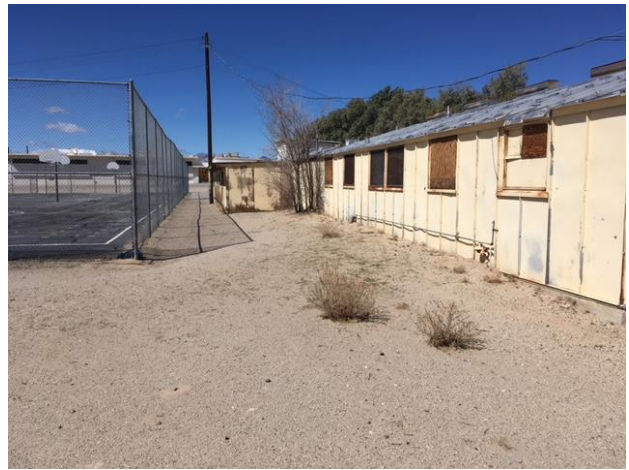
MJH54 – demolish metal & wood building; remove wood power pole; remove abandoned power line back to MJHPE building & disconnect at electrical panel; C.L. fence & basketball court to remain; smooth finish grade, no ponding
