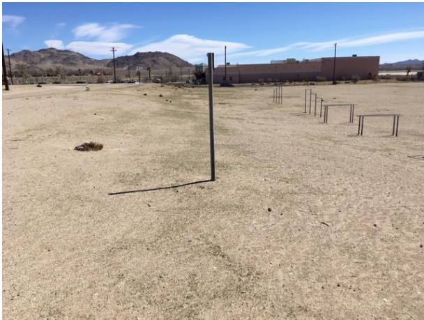
MJH56 – remove signage poles, footings, gymnastic pipes, footings, bf/compact; import clean fill dirt, smooth finish grade entire softball field west, no ponding
