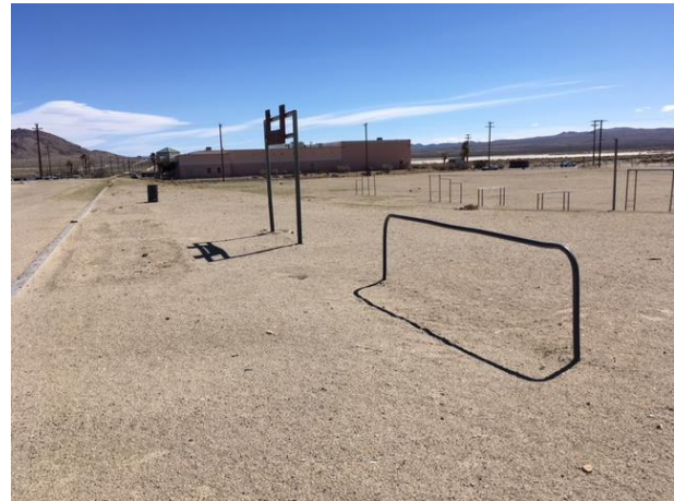
MJH56 – remove signage poles, footings, gymnastic pipes, footings, bf/compact; import clean fill dirt, smooth finish grade entire softball field west, no ponding
