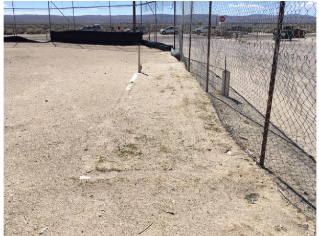
MJH55 – remove dugout pits, cap water line, remove riser, bf/compact
