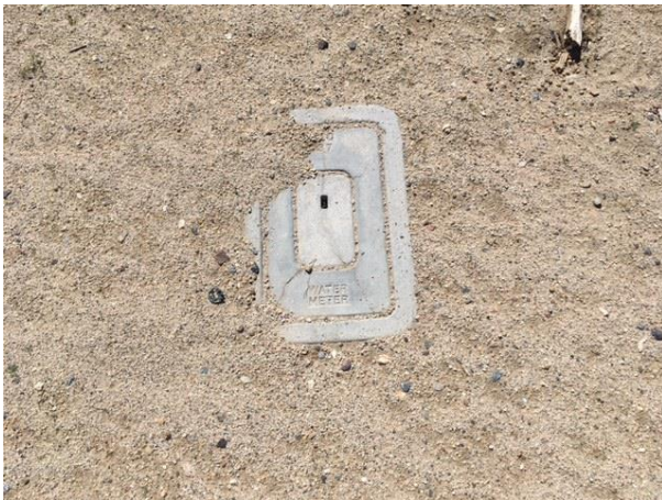
MJH58 – water meter to remain; protect in place
